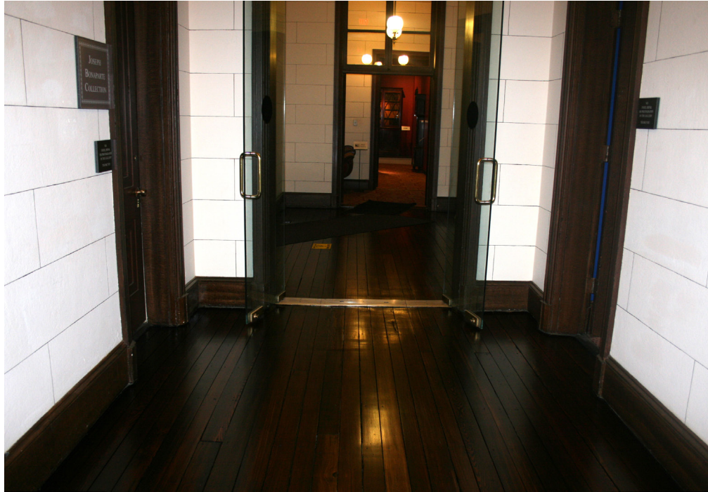
Re-finished floors in the front hall.
